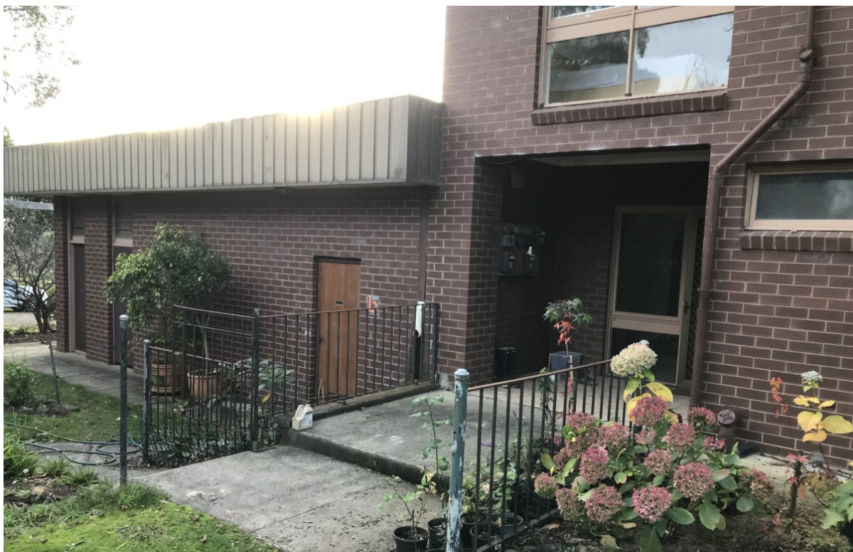
Photograph 2: Front of building – cellar door on left side, dwelling on right side
